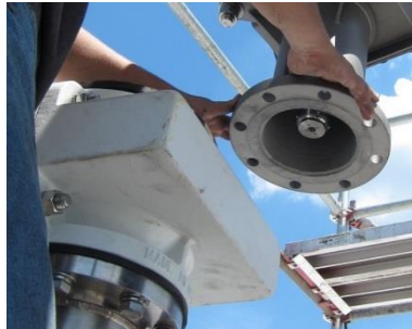
Figure 13 Aligning SI-7000 with mating flange
