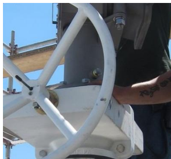
Figure 14 Installing mounting hardware
