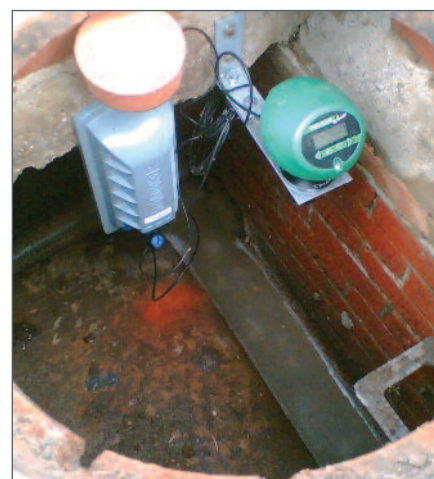
IMP MONITORING IN A CSO CHAMBER
